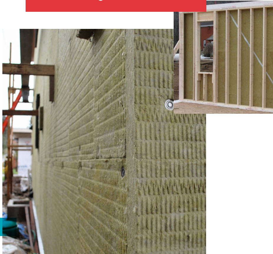
As an exterior insulation, ROCKWOOL Comfortboard™ 80 is fastened to the exterior OSB/plywood sheathing or structural stud wall and is designed to provide increased thermal performance to the building envelope
