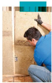
ROCKWOOL cuts quickly and accurately with a serrated knife, such as a bread knife, so you can easily achieve optimal fit around pipes, electrical boxes, wiring, ductwork and between studs and joists that are less than a standard width.
